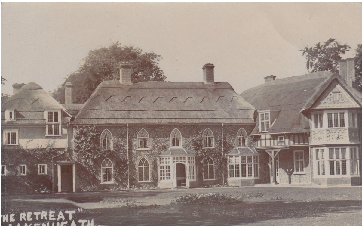
The Retreat before and after the extensions. Not far from Hall Drive a similar window shape can be seen. Where is it?
